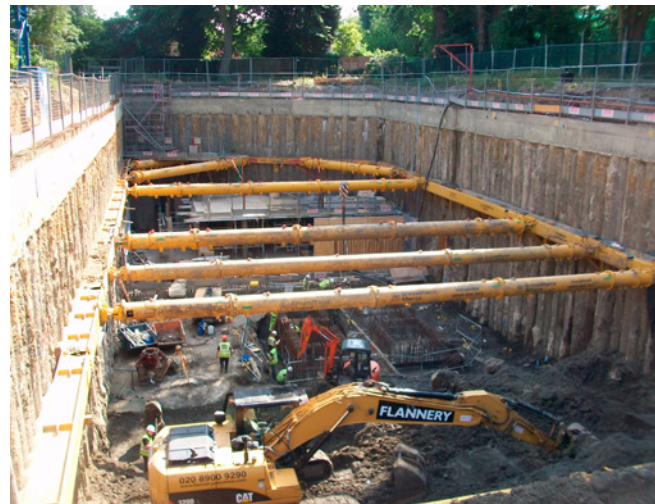
First slab steel fixing
