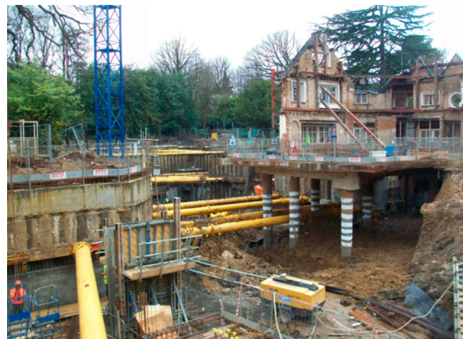
Work continues below and behind the existing facade
