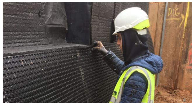
Platon Double Drain membrane improved drainage and protected the underlying self-adhesive waterproofing membrane.
