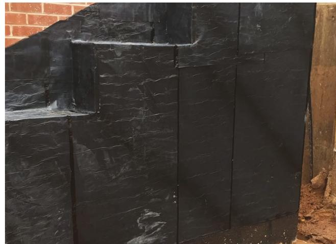
Triton's TWS EX-100 self adhesive membrane provided primary waterproofing to the retaining wall block work.
