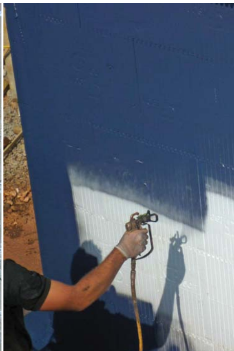
Figure 4: Spray-applied vapour membrane (see Figure 6).
