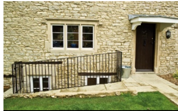
New light wells were created to front and rear of property
