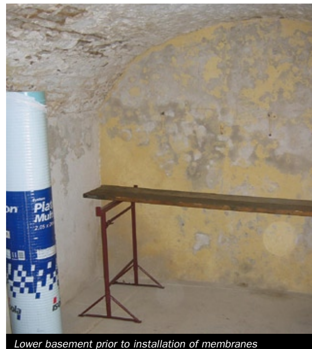
Lower basement prior to installation of membranes
