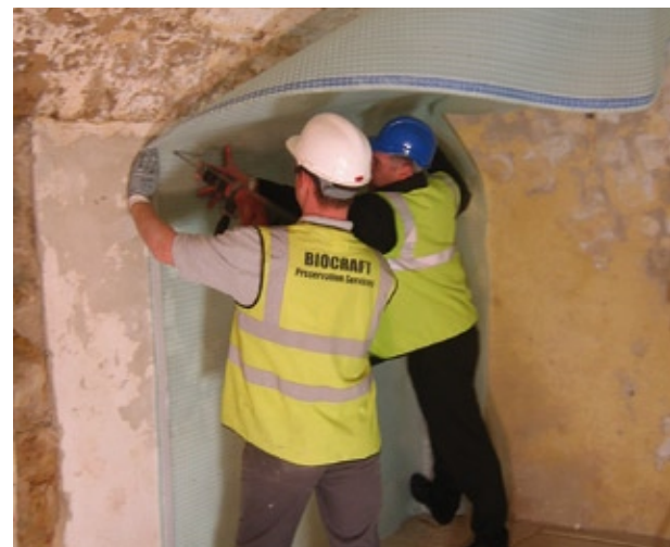
Installing Platon Multi
