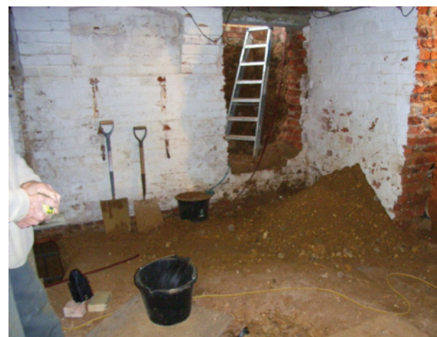
Basement before conversion
