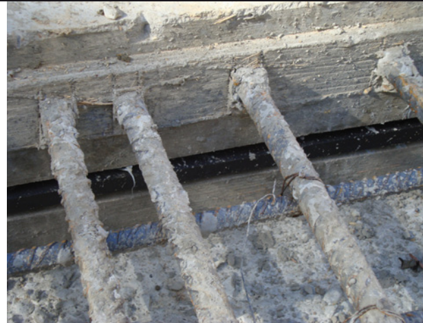
Sealed construction joint
