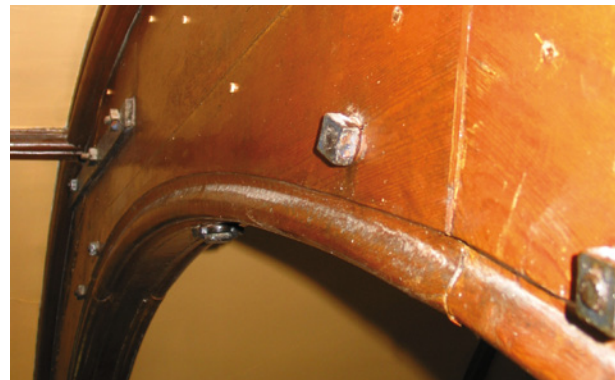
The pitch pine plugs were inserted by hand (standing slightly proud in photo) before being hammered flush with timber and stained
