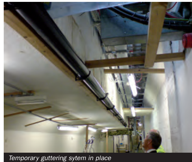
Render cracked and debonded in light wells
