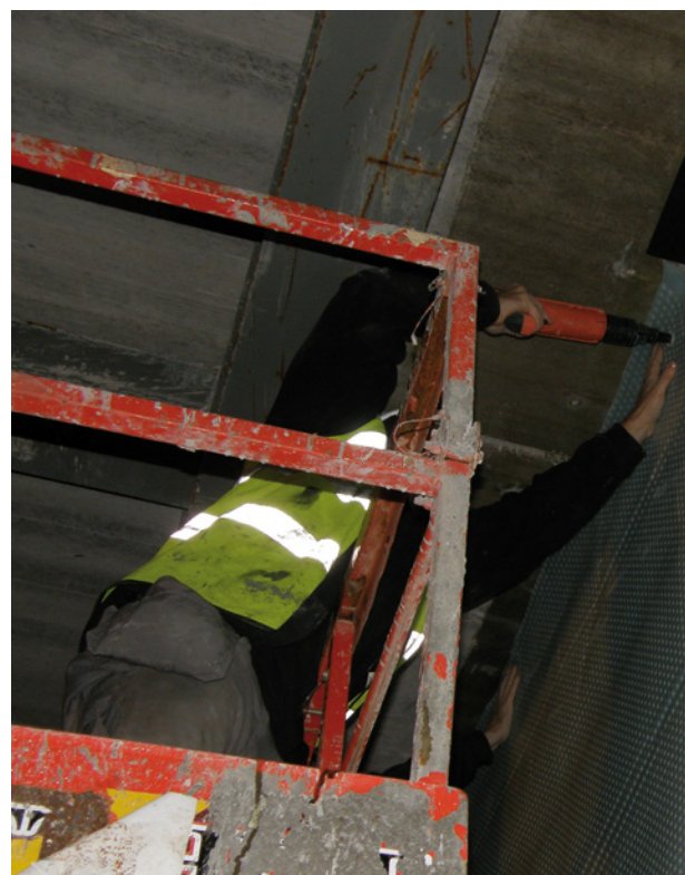
Platon Multi is fixed to the reinforced concrete walls
