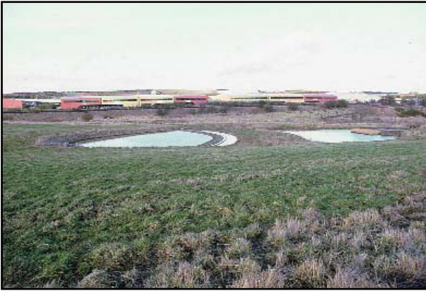
SUDS work in series: here a settling pond used to take out coarse sediment is followed by a filter strip
