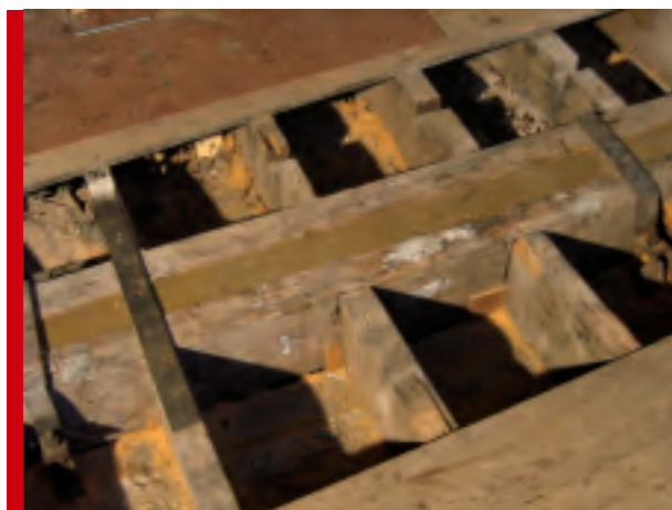
Beam strengthened with cured Trimol 36
