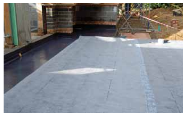
Platon Double Drain provided the secondary waterproofing layer
