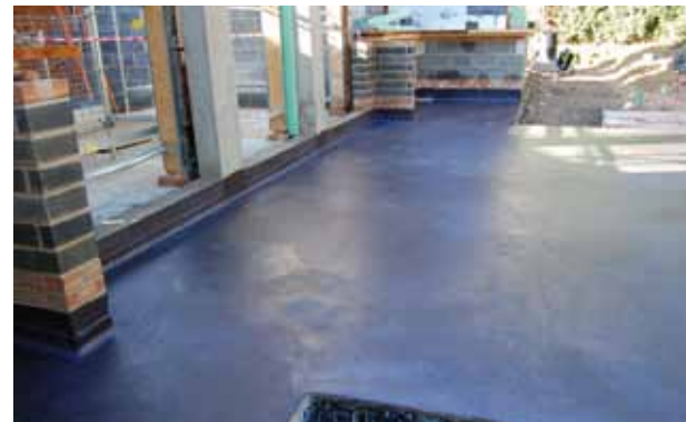
Two coats of TT Vapour Membrane were applied
