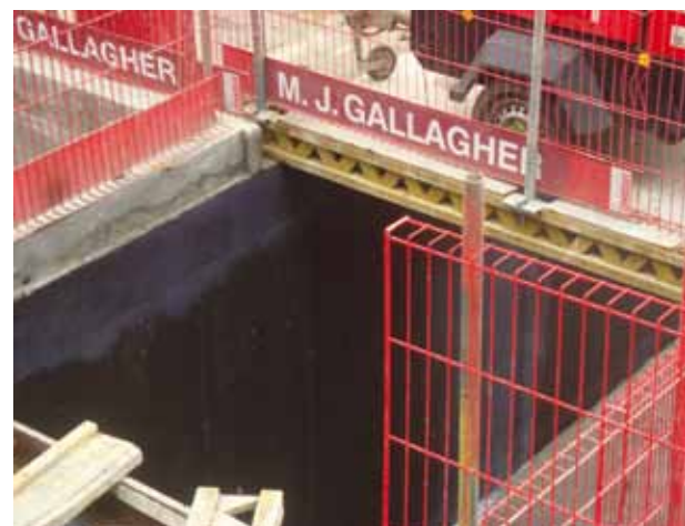
TT Vapour Membrane was used where it was impractical to install cavity drain membranes
