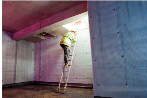
All perimeter walls were waterproofed with Platon Multi cavity drain membrane
