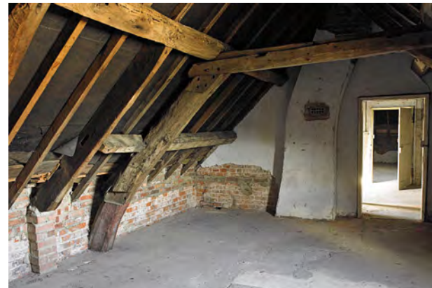
Timbers in the adjoining attics were also sprayed with Tritec 121
